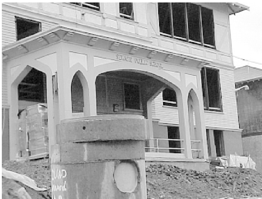
Seward under construction. November 1998
