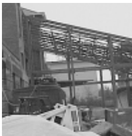
Seward LRC going up, January 1999.
