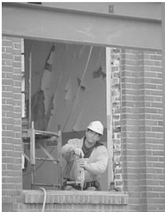
Seward brick building windows under construction, March 1999.
