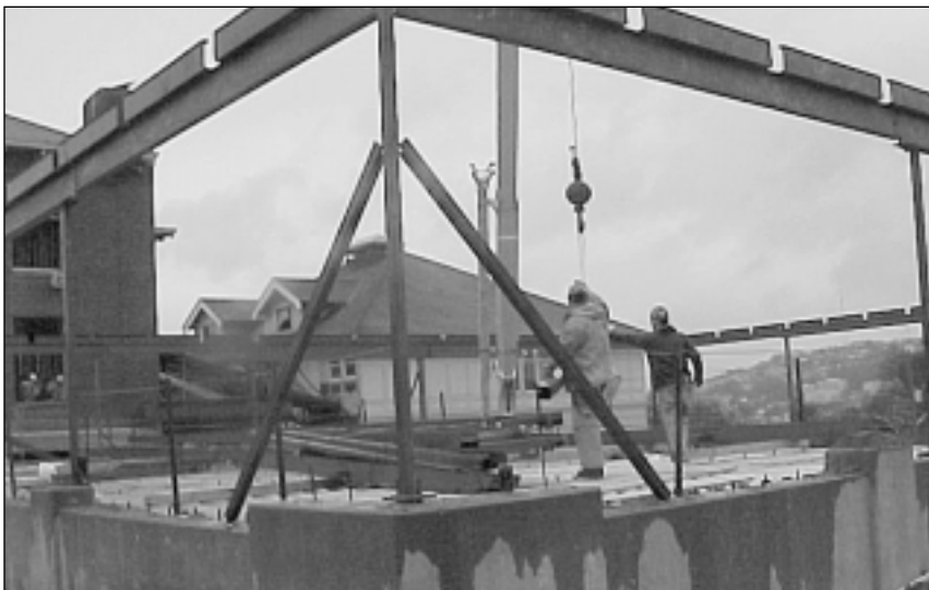
TOPS Gym at Seward under construction. March, 1999.
